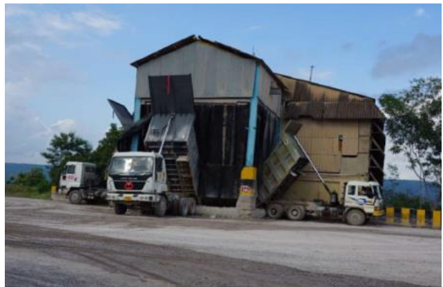
Rubber Curtains at Crusher Dump Hopper
