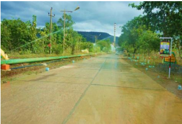
Fixed Water Sprinklers
