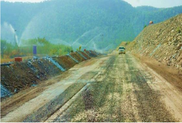
Water Sprinkling on Haul Road
