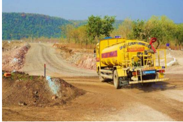
Dust Suppression at Internal Roads
