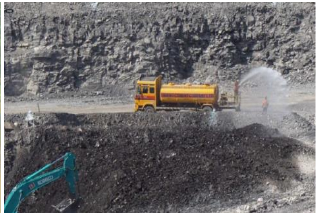
Muck Pile Wetting
