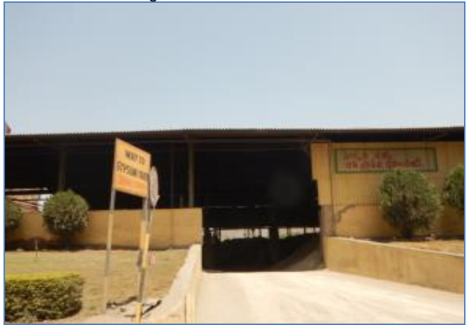
Gypsum Storage Shed
