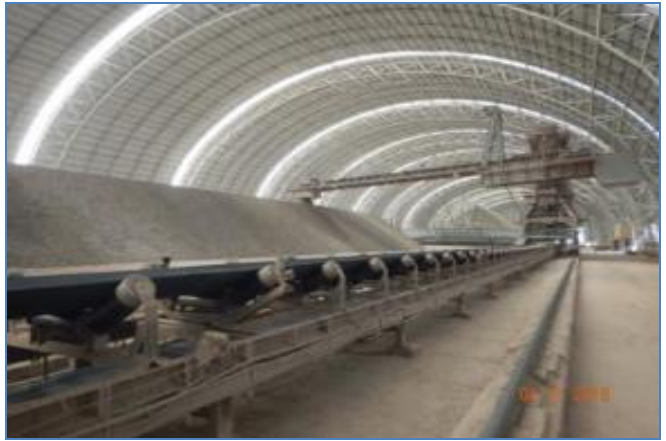
Limestone Storage Shed
