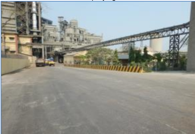
Internal CC Roads & Floorings
