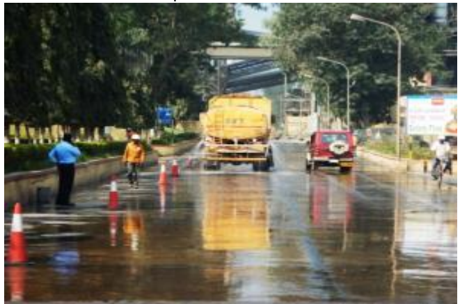
Water Spraying on internal roads
