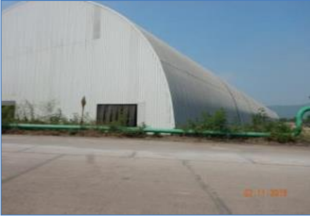
Coal Storage Shed
