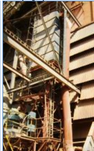
Bag filters at various material transfer points & silo top
