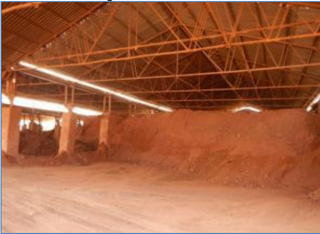
Laterite Storage Shed
