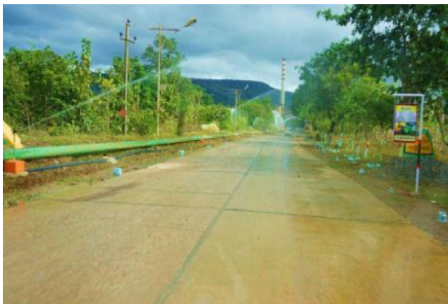
Fixed Water Sprinklers
