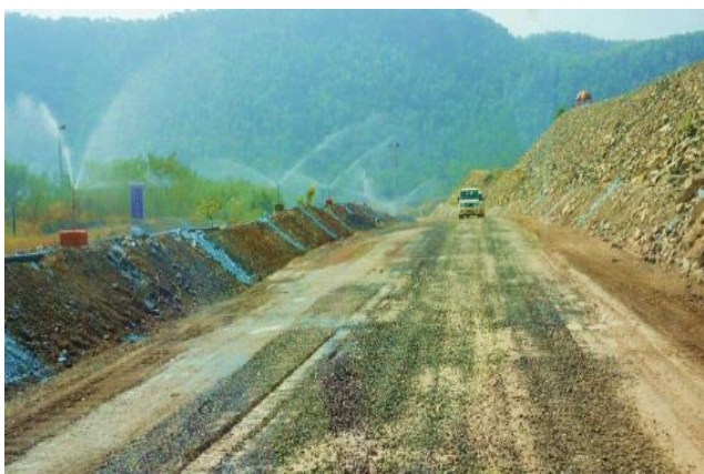
Water Sprinkling on Haul Road
