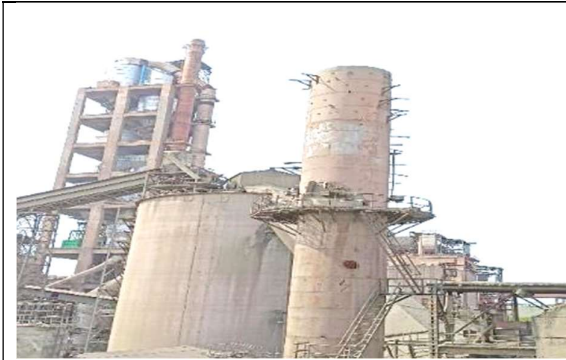
Kiln-3 RABH & Cooler-1 ESP stack
