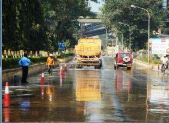
Water Spraying on internal roads
