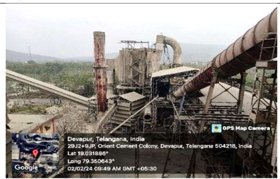
ESP for Clinker Cooler-3
