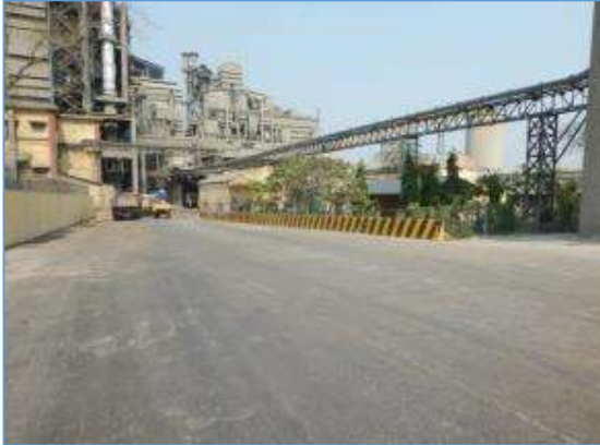
Internal CC Roads & Floorings
