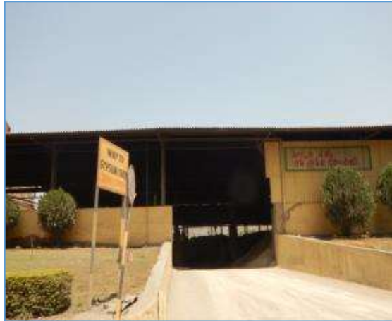
Gypsum Storage Shed
