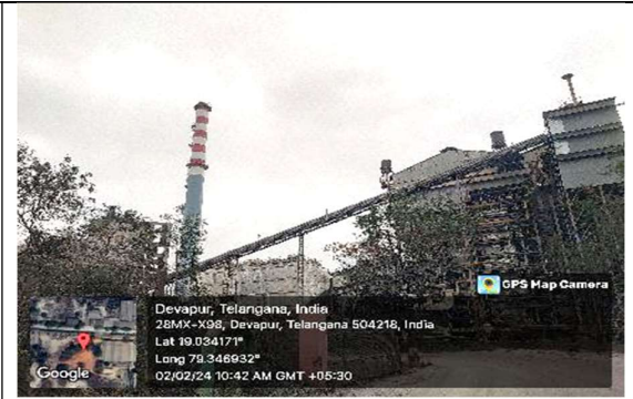
Stack of 2X25 MW CPP
