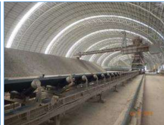
Limestone Storage Shed
