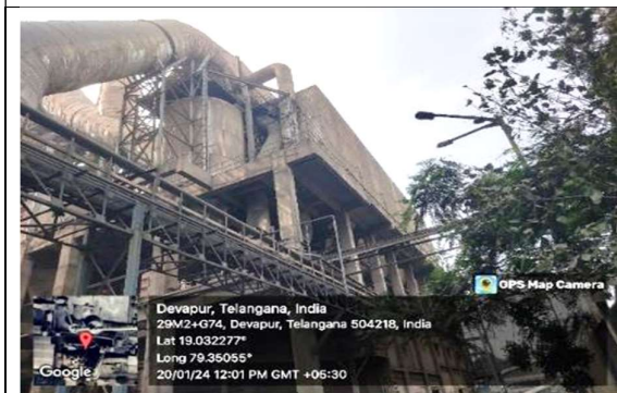
RABH for Kiln & Raw Mill -3
