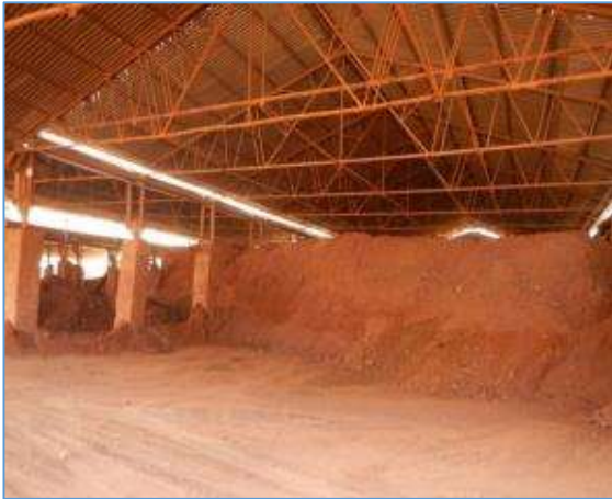
Laterite Storage Shed
