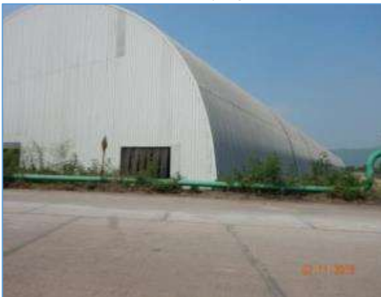
Coal Storage Shed
