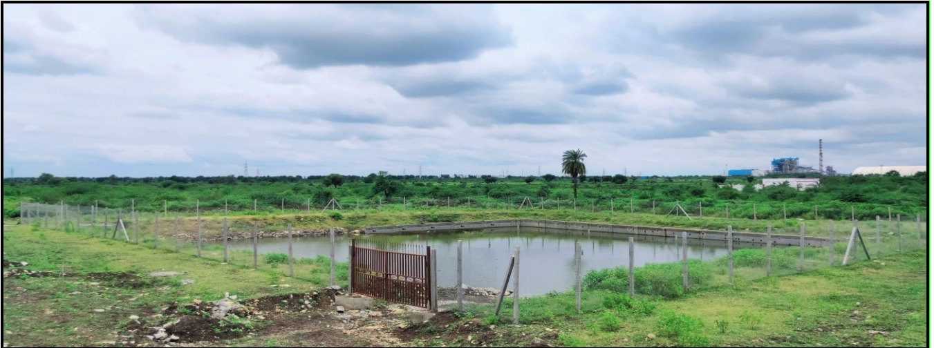
RAINWATER HARVESTING PIT cum SETTLING TANK
