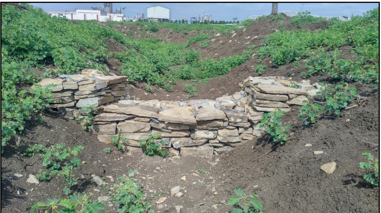
CATCHMENT/GARLAND DRAINS WITH RR DRY STONE BARRIERS
