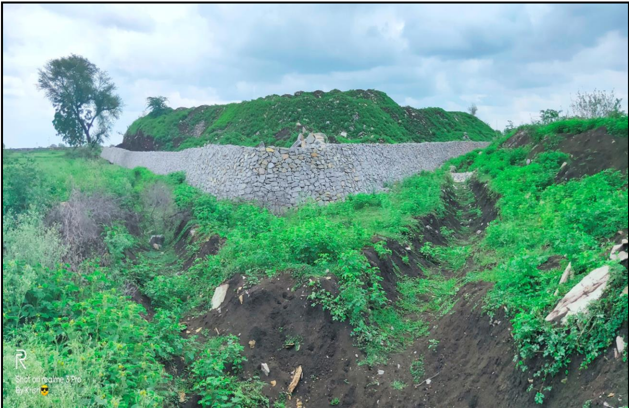
TOE WALL ALONG WITH GARLAND DRAIN AT BELOW THE TOPSOIL DUMP
