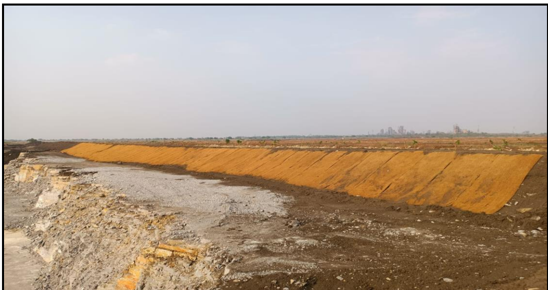
ECO-FRIENDLY GEO TEXTILE COIR MATT FOR SLOPE PROTECTION
