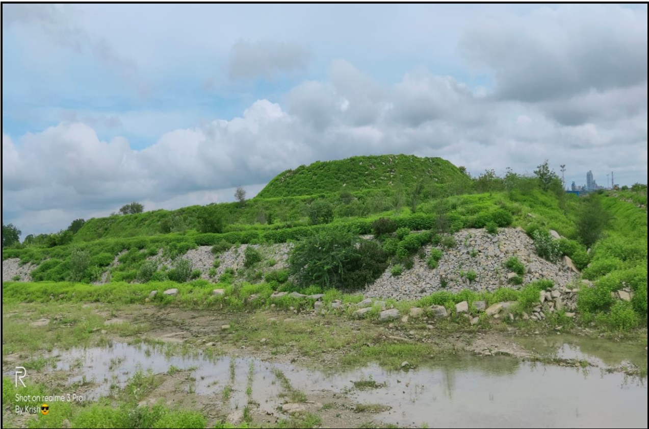
STONE PITCHING BELOW THE TOPSOIL DUMP
