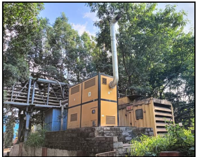
Retrofitted Emission Control Devices for the DG sets
