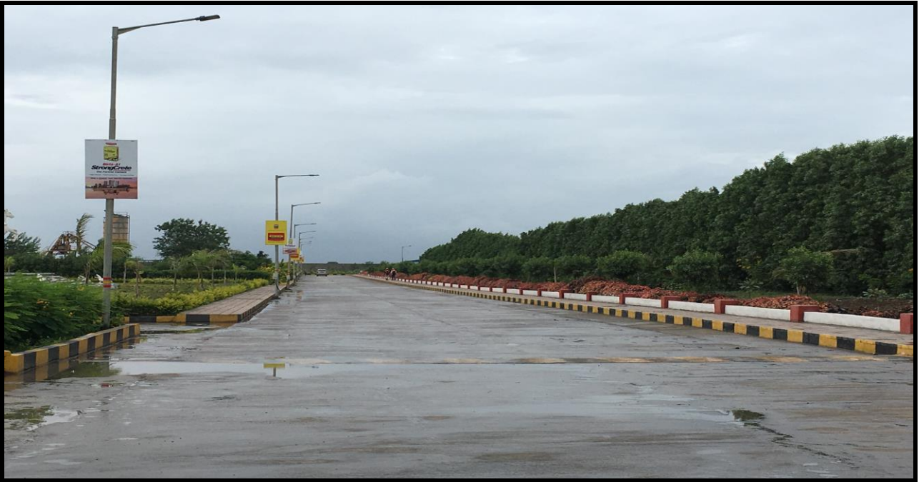
Concrete road inside the plant to avoid fugitive dust
