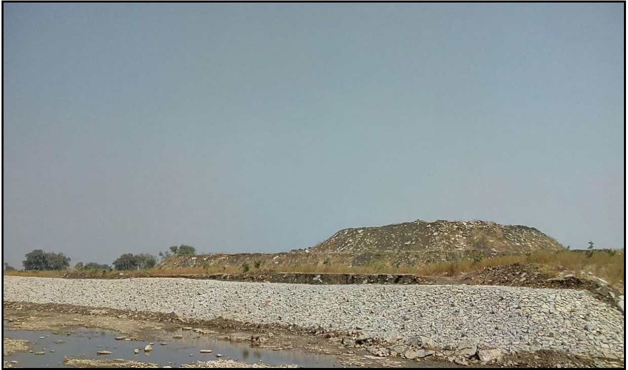
BC Soil Dump with Protection Wall
