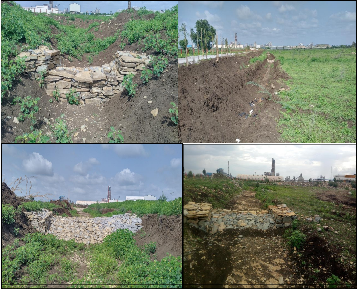
Catchment Drains with RR Dry Stone Barriers
