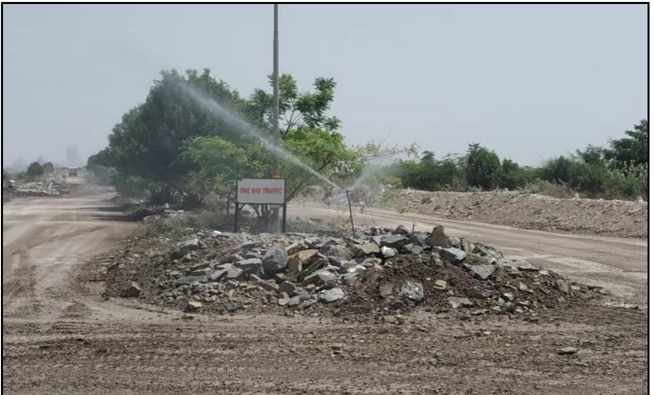
Water sprinkler along the Haulage road
