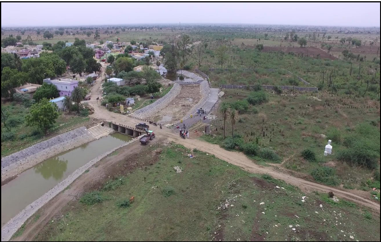
STONE PITCHING ALONG THE NALA BANKS
