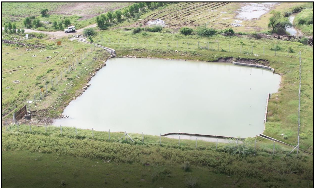
RAINWATER HARVESTING PIT cum SETTLING TANK
