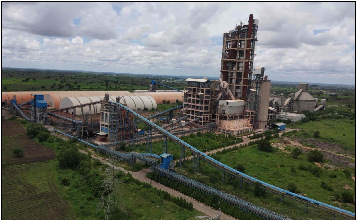
Belt Conveyors are fully covered
