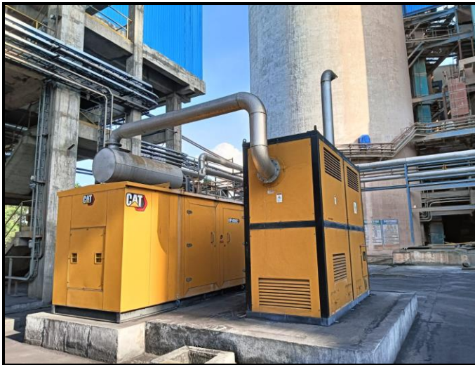
Retrofitted Emission Control Devices for the DG sets
