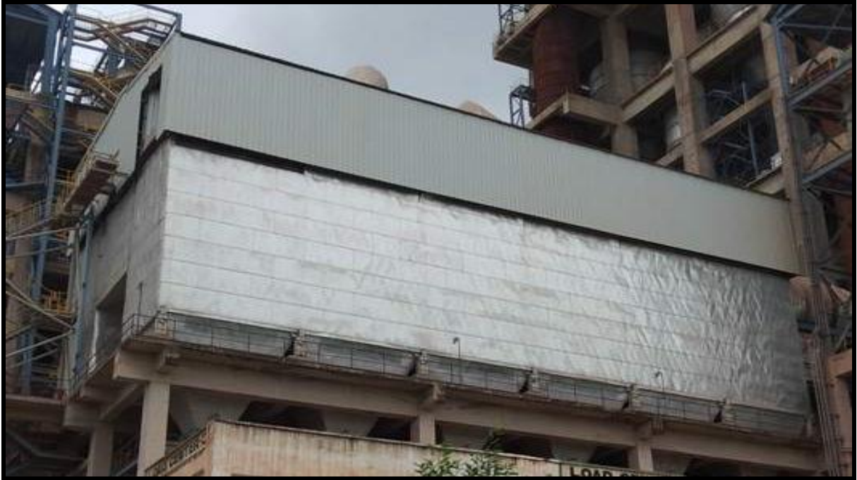
ESP for Cooler and CPP
