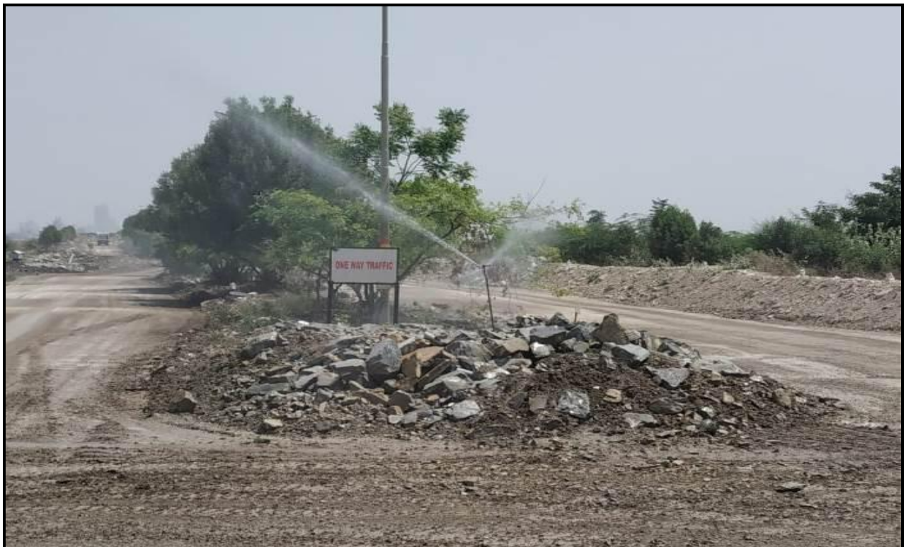
Water sprinkler along the Haulage road
