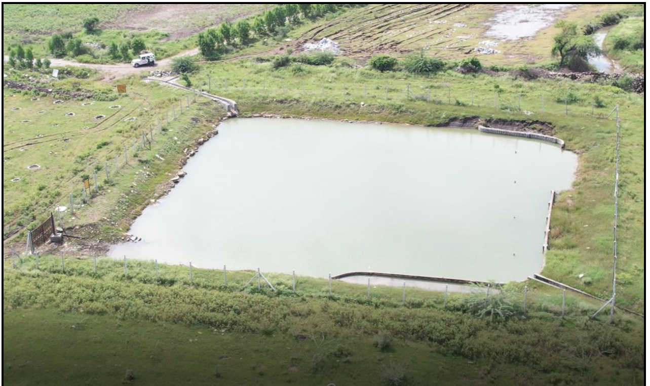
RAINWATER HARVESTING PIT cum SETTLING TANK
