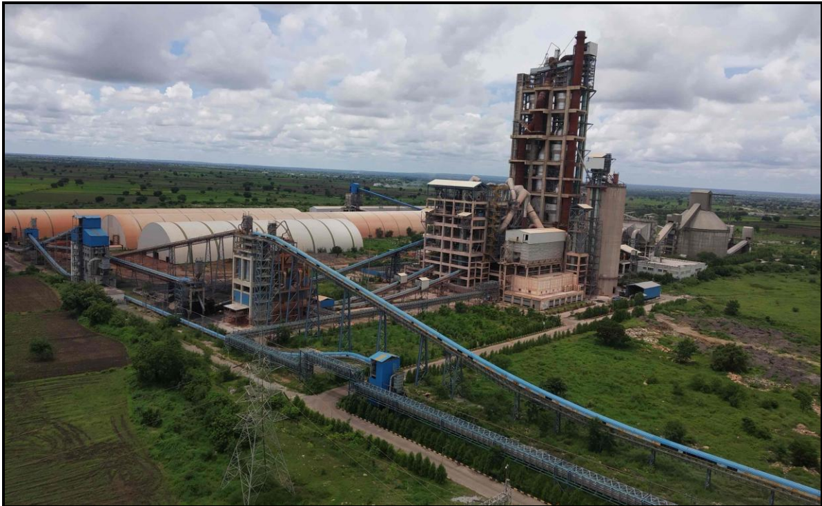
Belt Conveyors are fully covered
