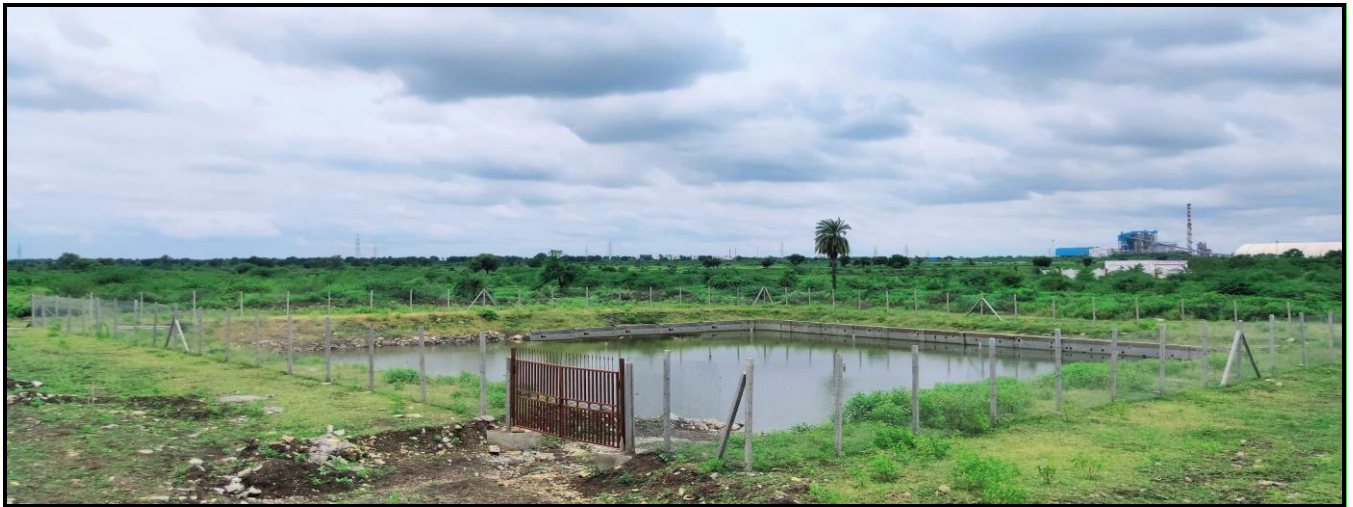
RAINWATER HARVESTING PIT cum SETTLING TANK
