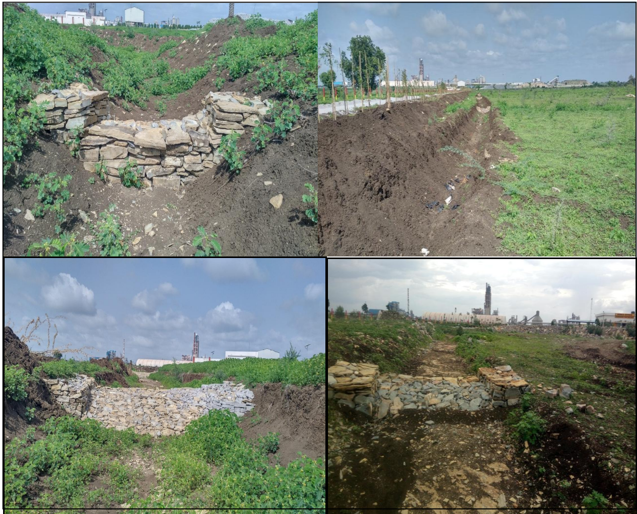
Catchment Drains with RR Dry Stone Barriers
