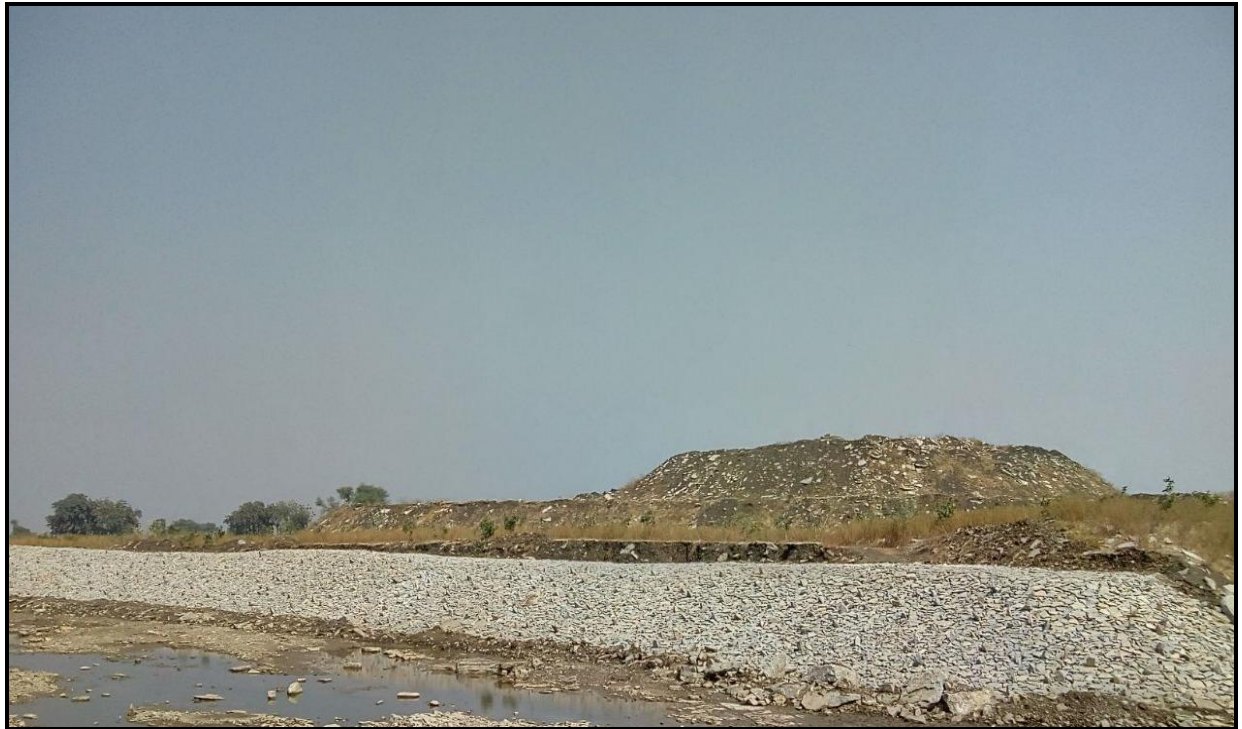
BC Soil Dump with Protection Wall
