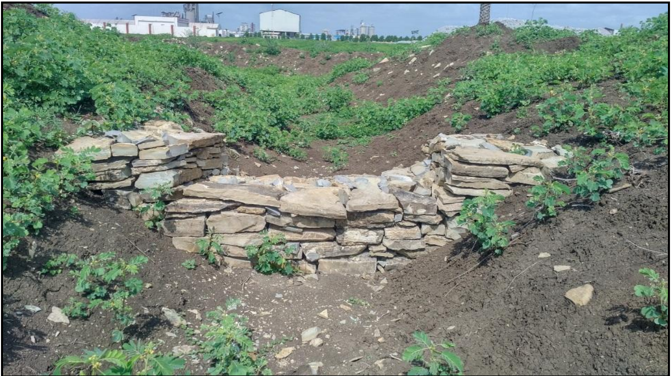
CATCHMENT/GARLAND DRAINS WITH RR DRY STONE BARRIERS
