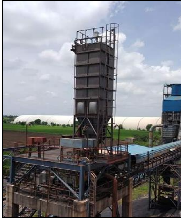
Bag Filters at all transfer points
