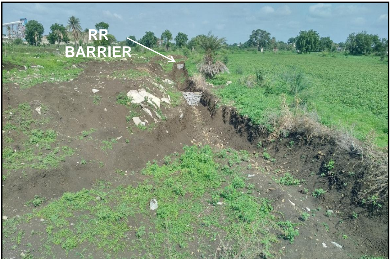
Garland drain with RR barrier
