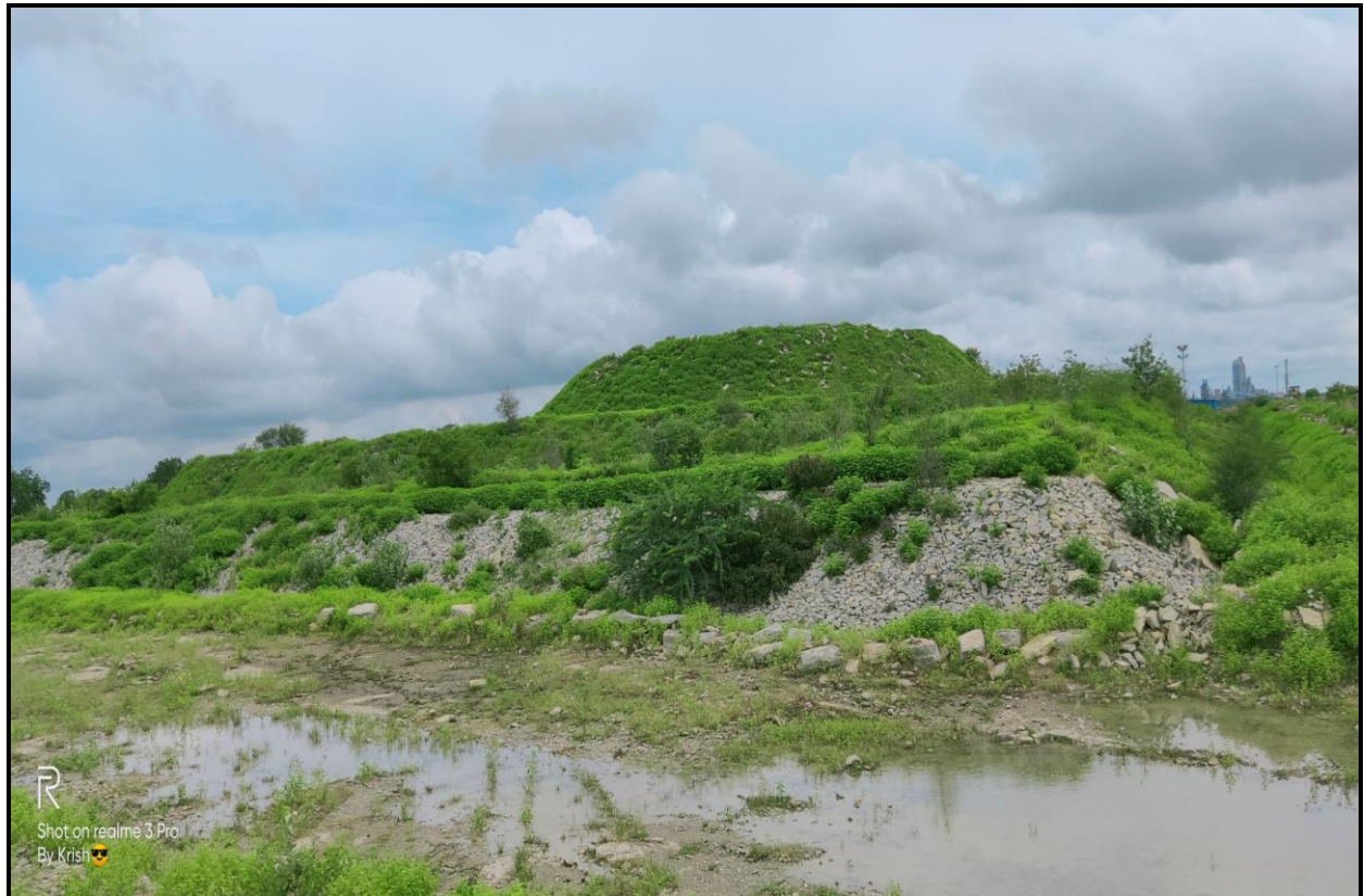
STONE PITCHING BELOW THE TOPSOIL DUMP
