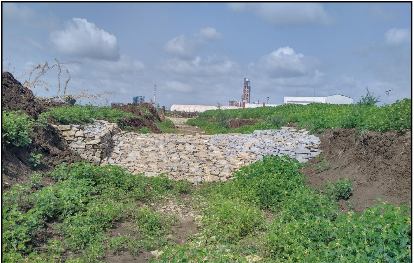
CATCHMENT/GARLAND DRAINS IN MINES AREA
