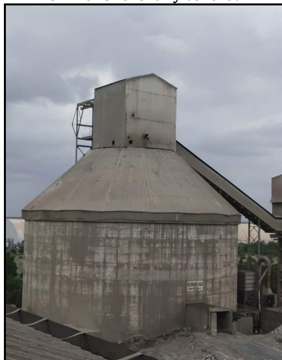
Clinker Silo is fully covered
