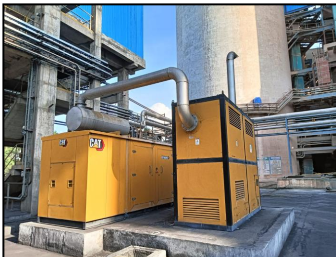
Retrofitted Emission Control Devices for the DG sets Details of Environmental Cell
