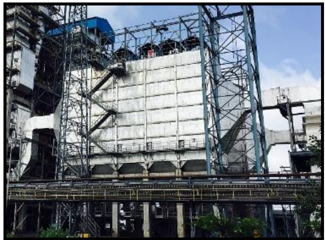
ESP for Cooler and CPP
