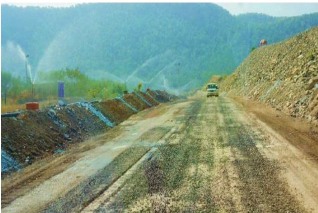
Water Sprinkling on Haul Road
