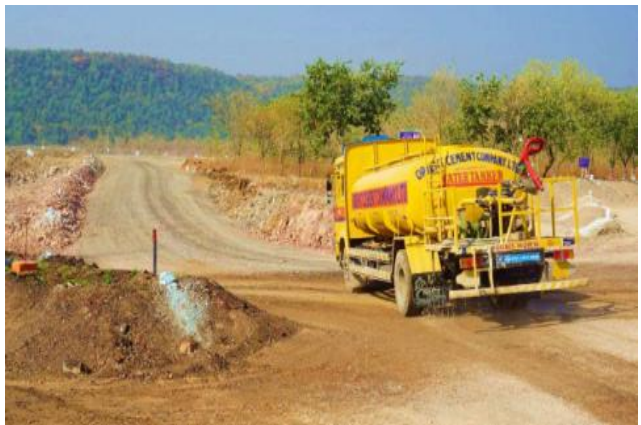
Dust Suppression at Internal Roads
