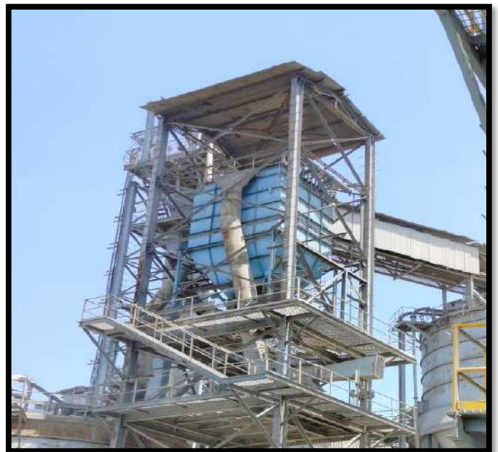
Fly Ash Silo Bag Filter
