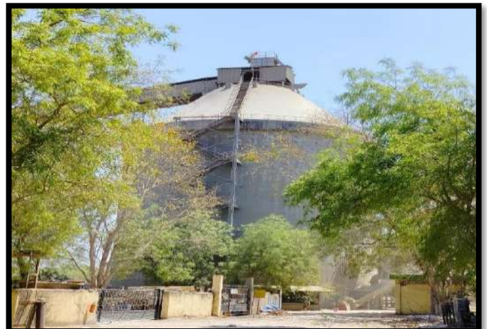
Clinker Storage in Closed Silo
