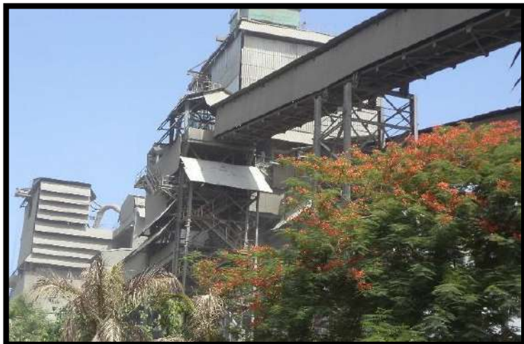
Figure 1: Closed Conveyors System
