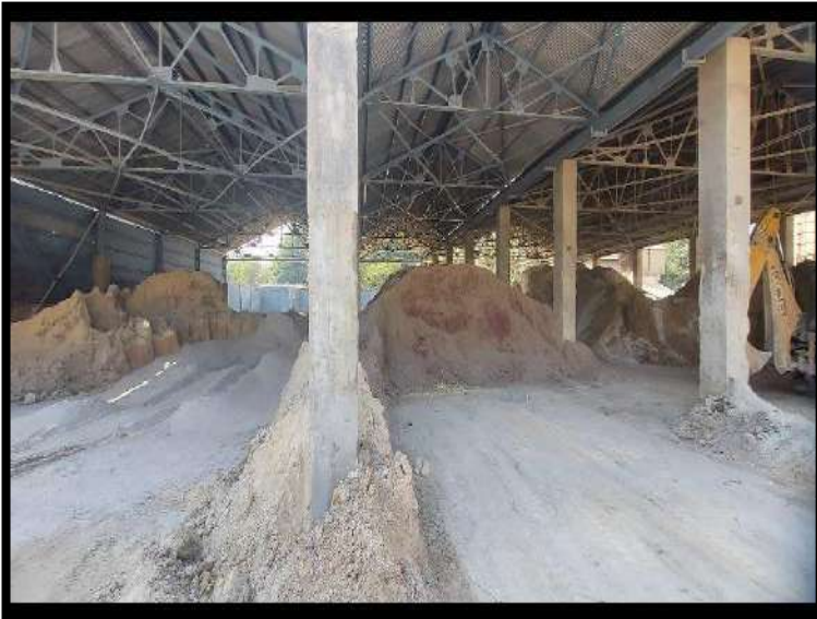
Figure 6: Covered Shed along with concrete floor for Gypsum Storage
