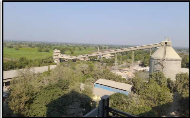
Closed Conveying System
