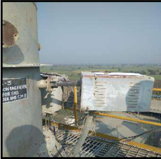
CEMs System installed at Cement Mill – 1 & 2 Stacks
