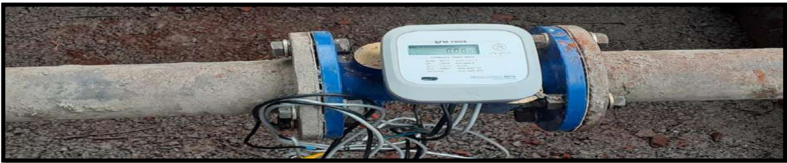
Digital Water Flow Meter at Water Withdrawal Points
