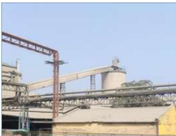
Closed Conveying System
