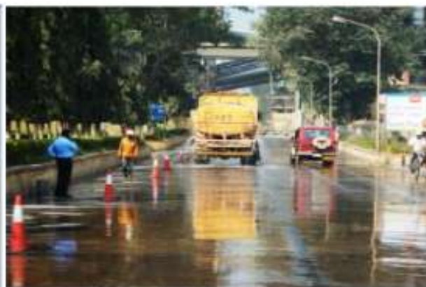
Water Spraying on internal roads
